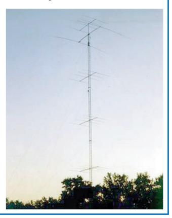
$40M\colon 2el$  Cushcraft yagi at 26m. On 75/80 and 160 I use Inverted V's and two bevarages NW and NE.
